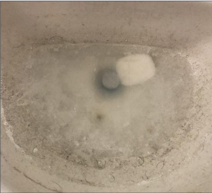
Dirty, clogged bathroom sink with hair
