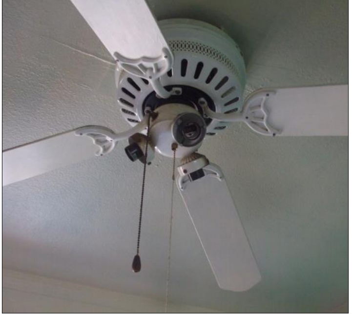
Ceiling fan missing lightbulbs; no other lighting in bedroom Home 21
